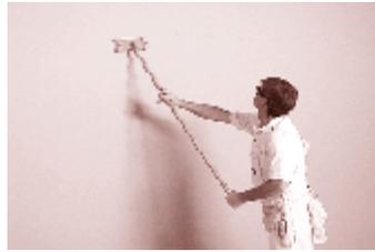
**Tip:** In order to reduce the amount of work needed to prepare your wall, mark the rectangle where EganWall is to be installed. Concentrate on bringing this area to a 'Level 5' finish, rather than the entire wall.
